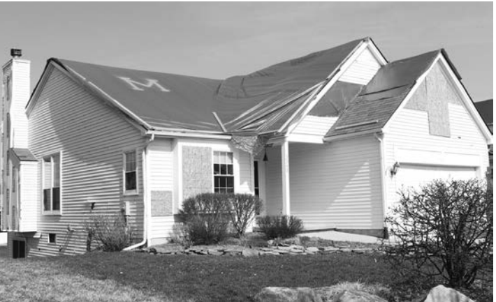
Tarps cover the damaged roof of a home in Dexter to protect it from the weather.
